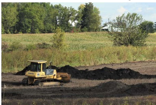
Earth moving—shaping the contours and depressions, creating "potholes" and emergency spillway Photo by Randy Lehman
