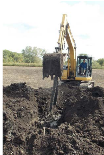
Removal of drainage tile Photo by Ken Brunswick
